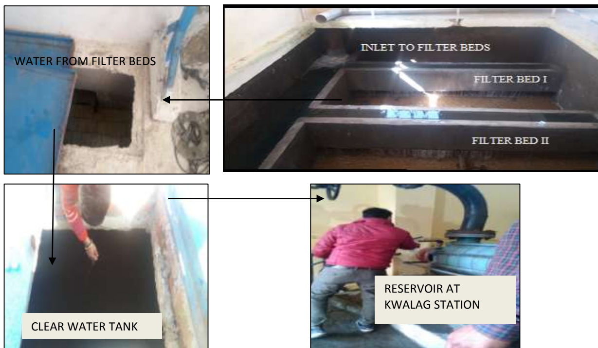
Fig 3.2 Various sampling points at different stages of water supply from Ashwani Khud WTP
