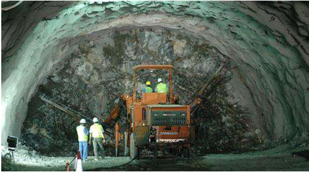
Fig 3.4 Rock Bolt supporting
