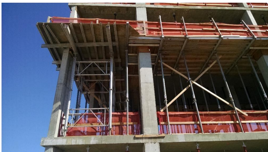
FIGURE 4.7 Use of guard rails
