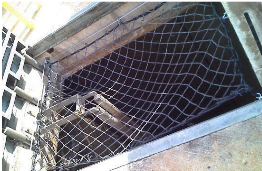
FIGURE 4.6 Use of safety nets
