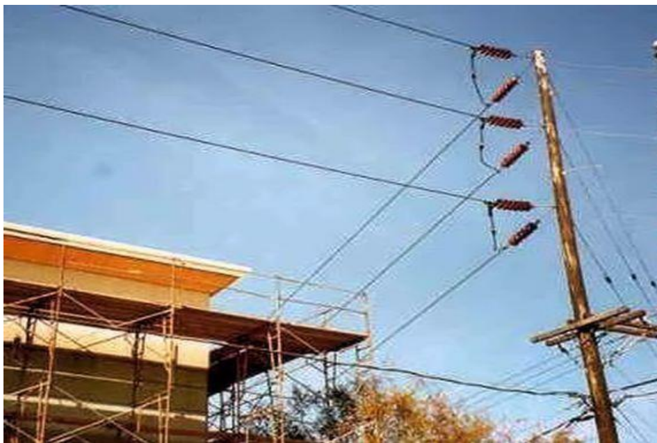
FIGURE 2.1 Electrical energy sources at construction worksites are power lines
