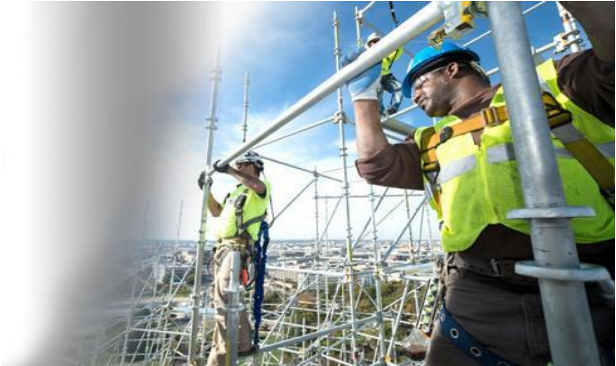
FIGER 4.1 working at elevated place
