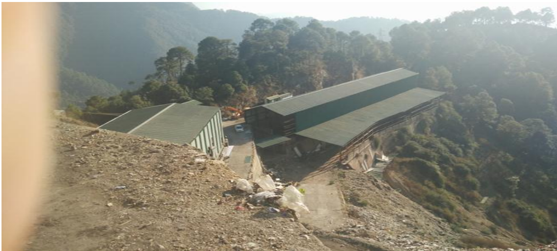
Figure 1.2 Existing Landfill site and waste to energy plant site at Bhariyal Shimla
