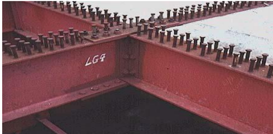
Figure 1.3 Shear Connectors
