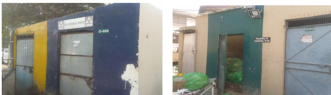
Plate 5.18: A view of Lockable Shacks at the Backyard of IVY Hospital.
