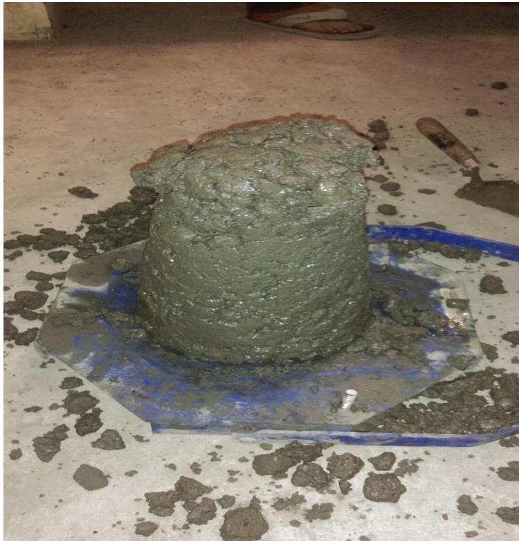
Fig no. 3.5 Slump test
