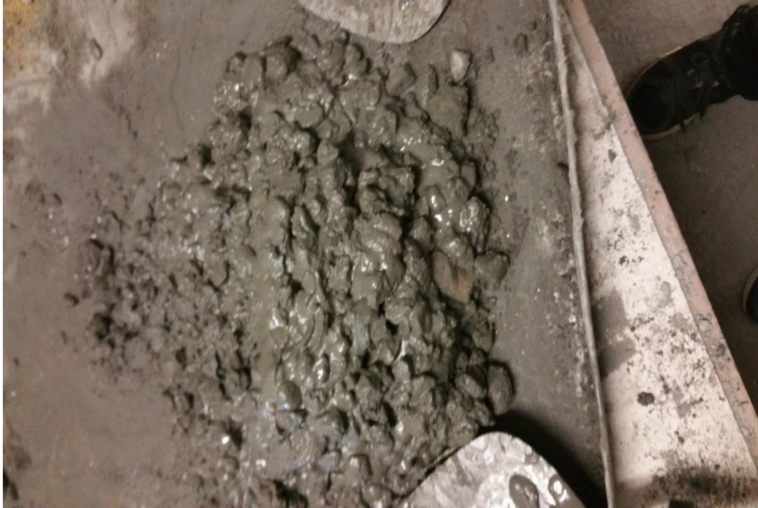
Fig no. 3.3 Mixing of concrete
