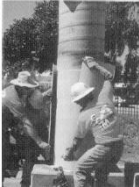
Figure 34: Confining system based on pre-fabricated FRP elements
