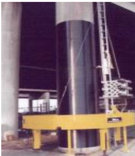
Figure 35: Automatic RC column wrapping
