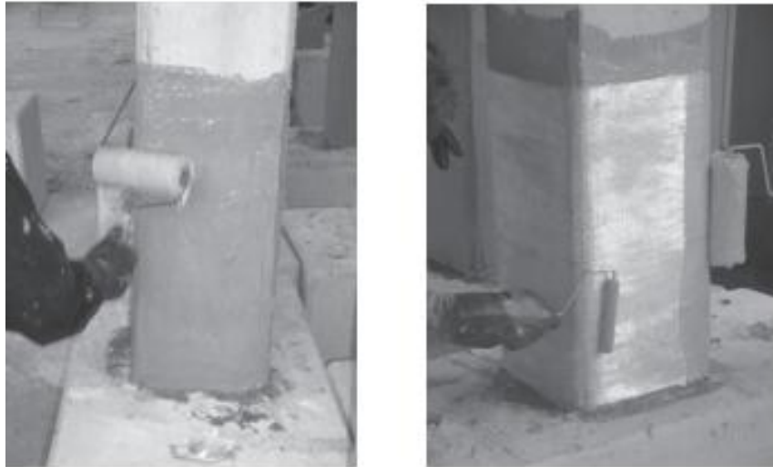
Figure 33: Wet up confining FRP system
