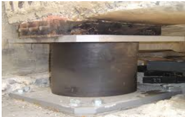
Fig. 1.2 Lead Rubber Bearing
