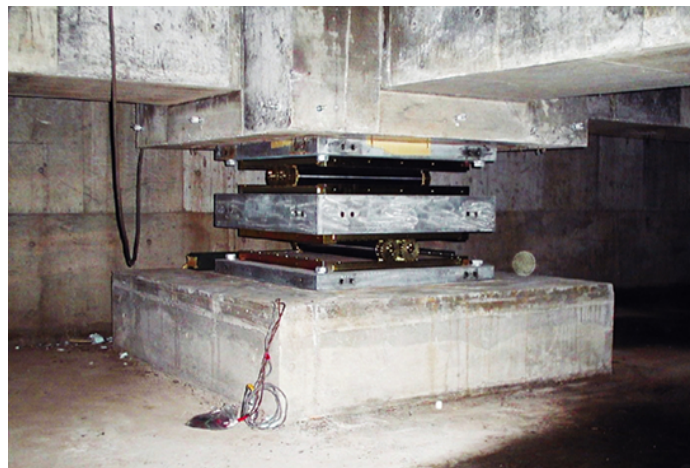
Fig 1.4 Simple Roller Bearing
