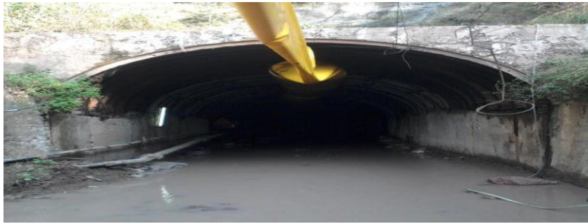
Fig 4.4 Adit at Chakhran Village
