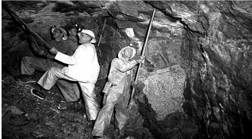
Fig 7.2 Manual Scaling of the Tunnel
