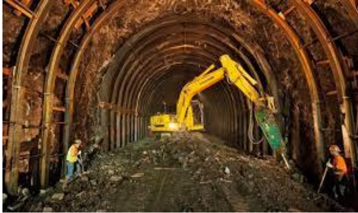
Fig 7.1 Providing Steel Ribs at the portal
