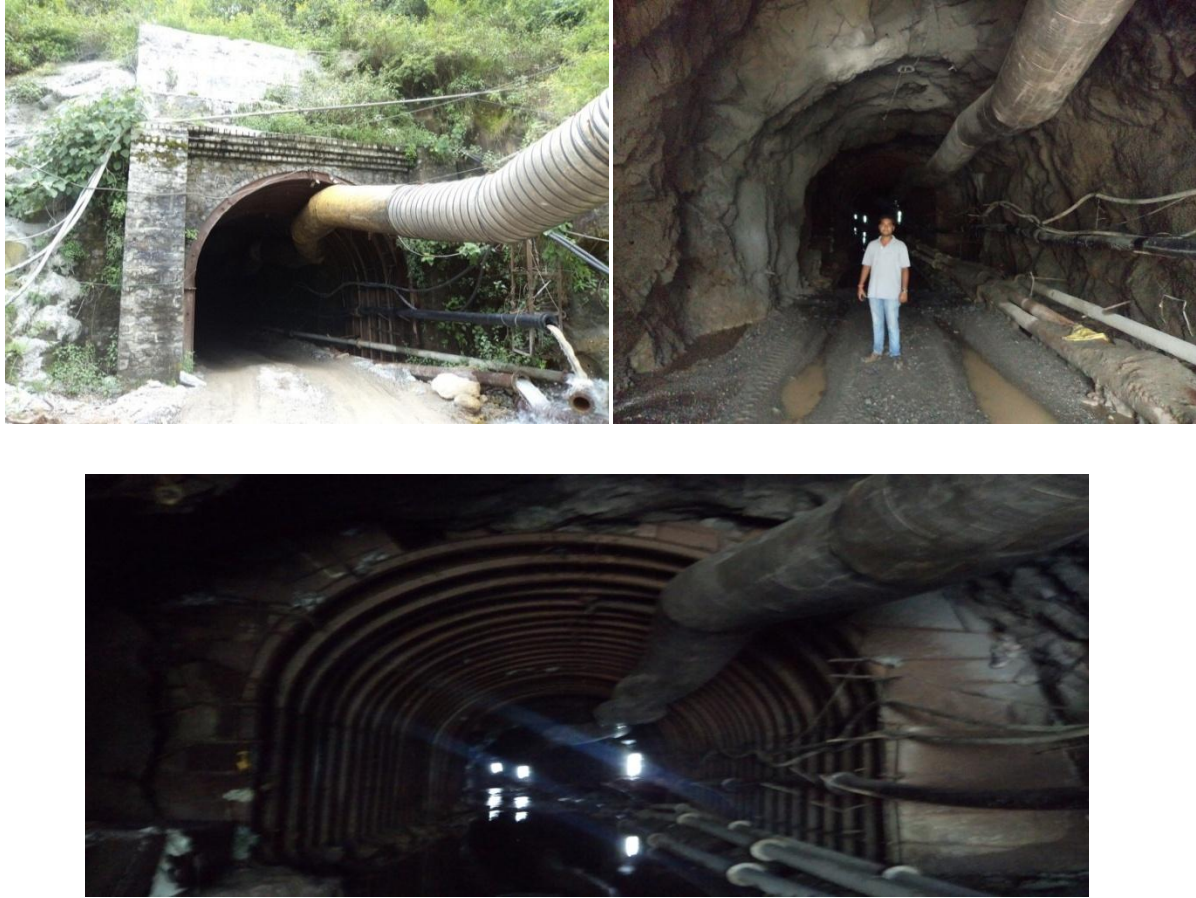
Fig 3.1 Head Race Tunnel
