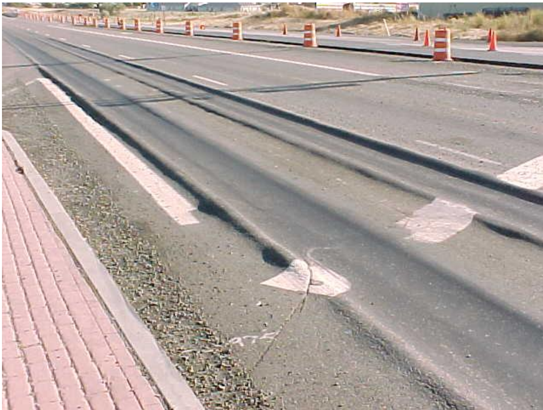
Fig. 2-Pavement Deterioration (Rutting)
