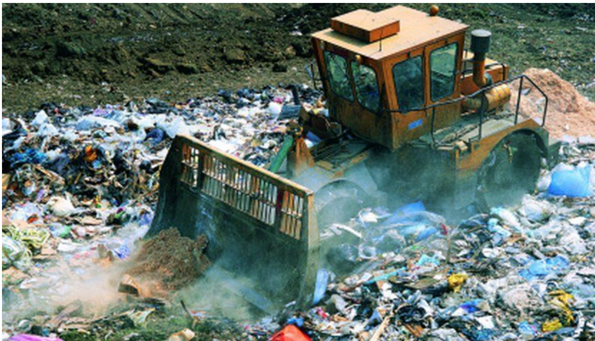
Fig.2.1: JCB clearing the MSW on the Landfill Site
