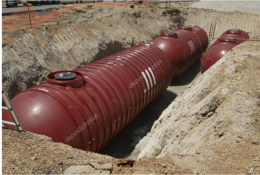
Figure2 : underground storage tank
