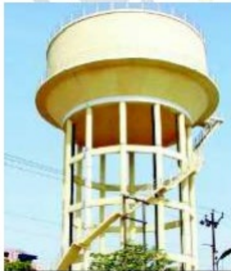
Figure (6): Intze type Water tank
