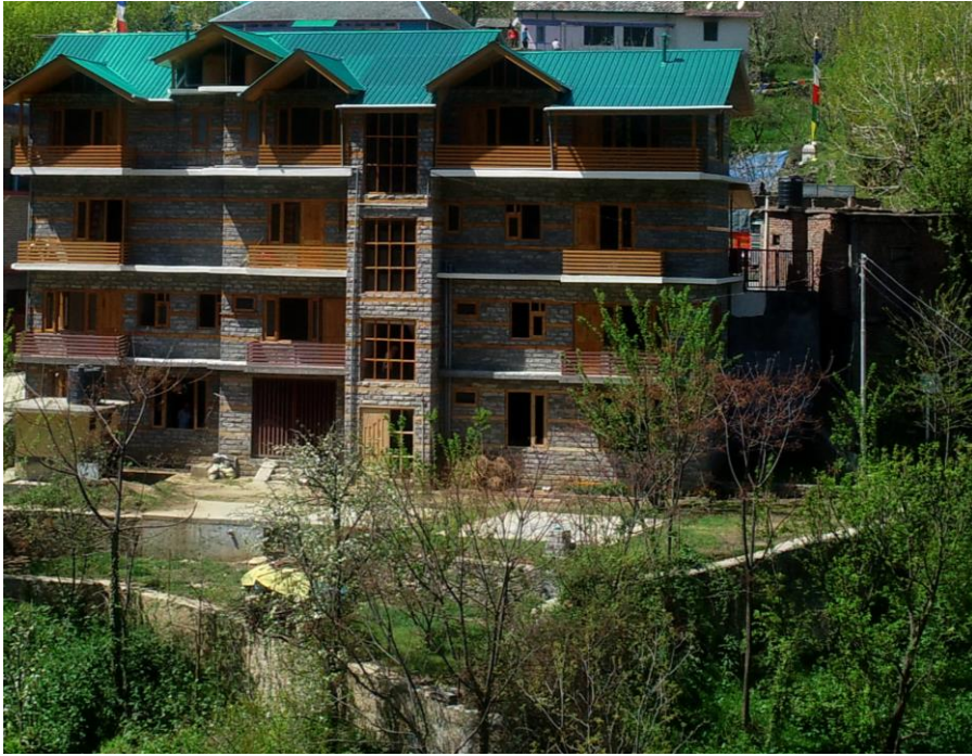
Figure 15: building at kullu
