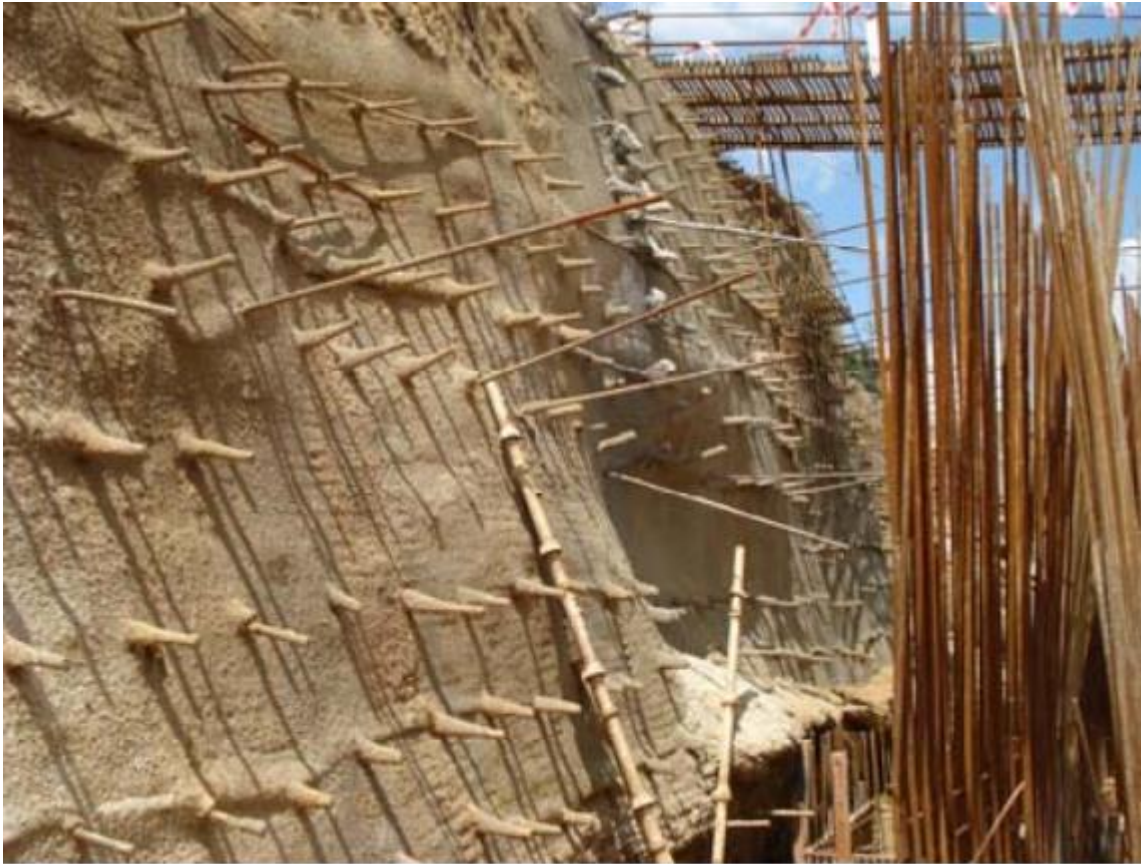
Fig.2. 33 Soil Nailed Wall [62]
