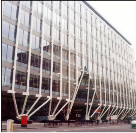
(a) Fleet Place House (London, UK)
