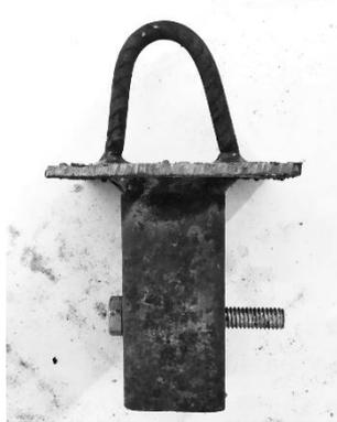
**Figure 3.7** Pile cap for single pile
