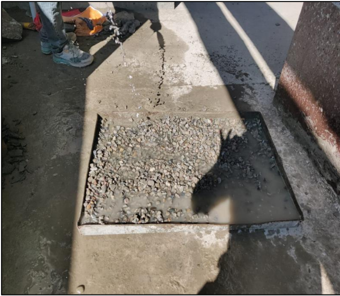
Figure 7: Water washing the aggregates
