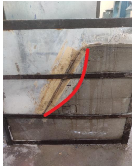
Figure 4.9 (b) Side view of slope after failure
