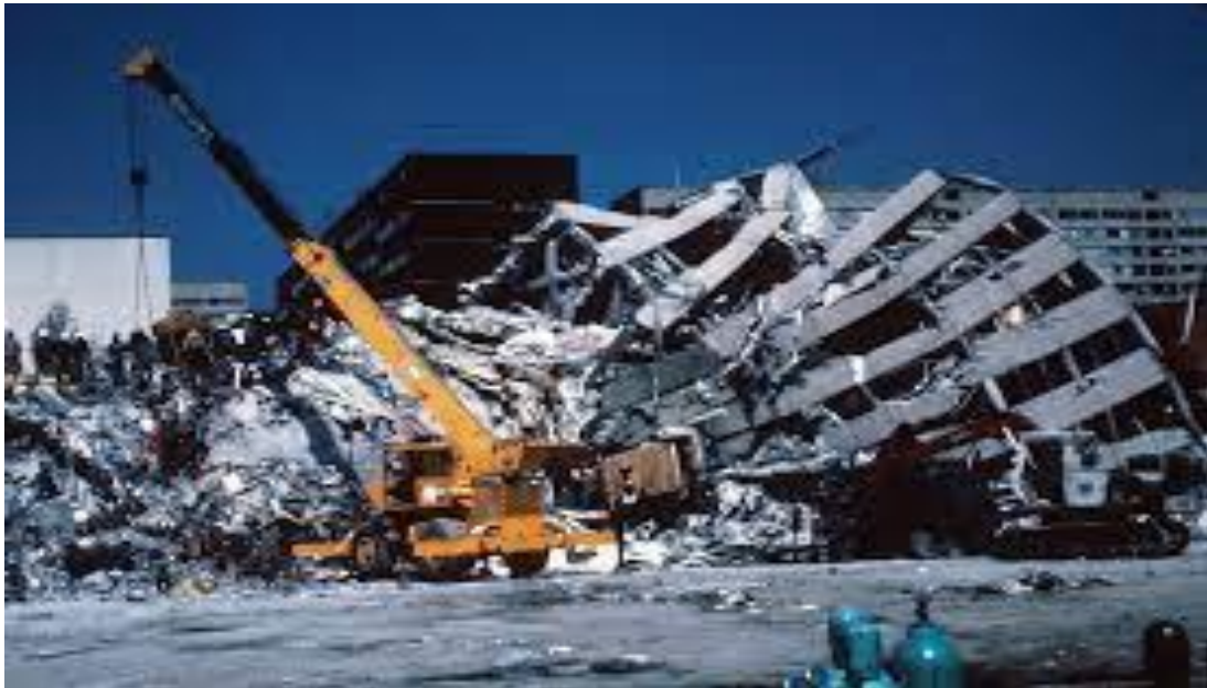
Figure 5 Collapse of Juarez Hospital
